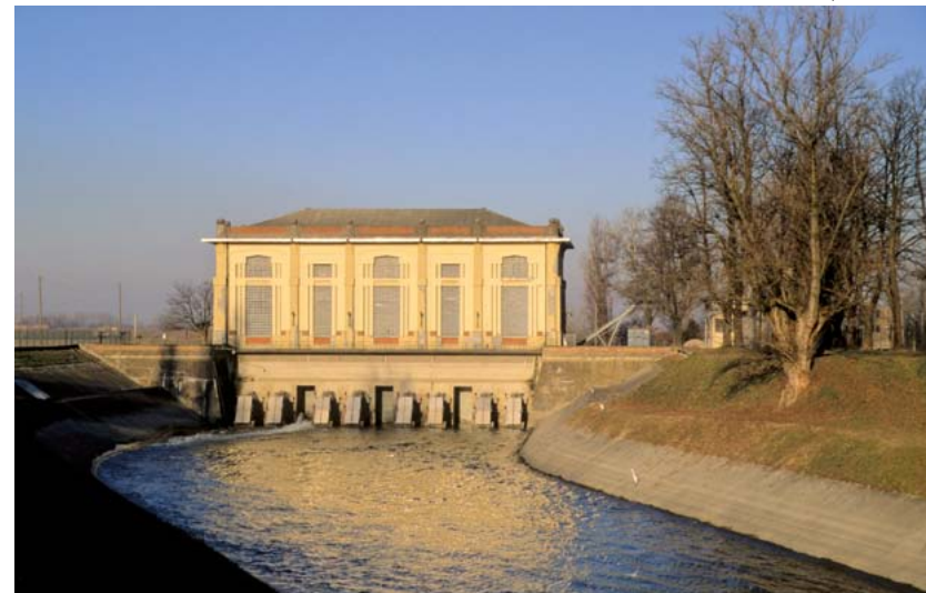
Santa Bianca, water works
